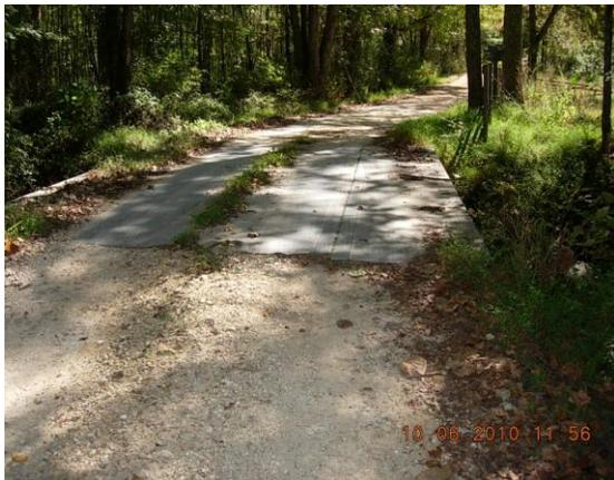
Figure 1: Bridge built from mercury fuel cells
